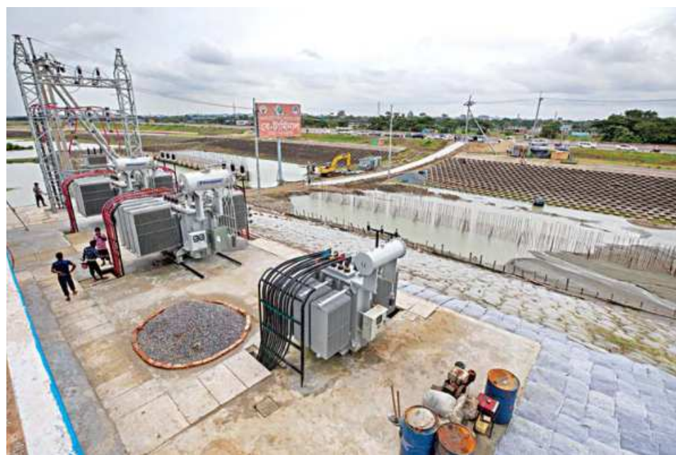
Construction work for Bay Terminal, a long-awaited mega expansion project of the Chattogram port, has gained momentum as the government has set 2024 to start operation of the terminal. The photos were taken yesterday.
