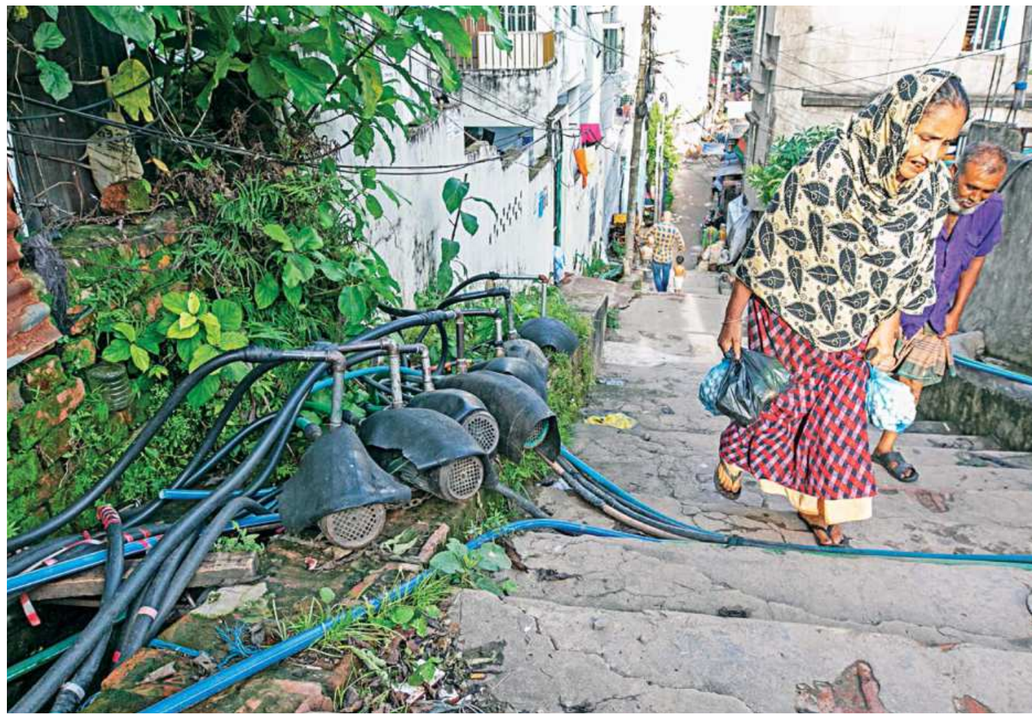
As the pressure of supply water is low in the hills of Motijharna in Chattogram city, some people install illegal pumps to fill the tanks of their homes. This, however, deprives their neighbours who chose not to indulge in the illegal activity.
