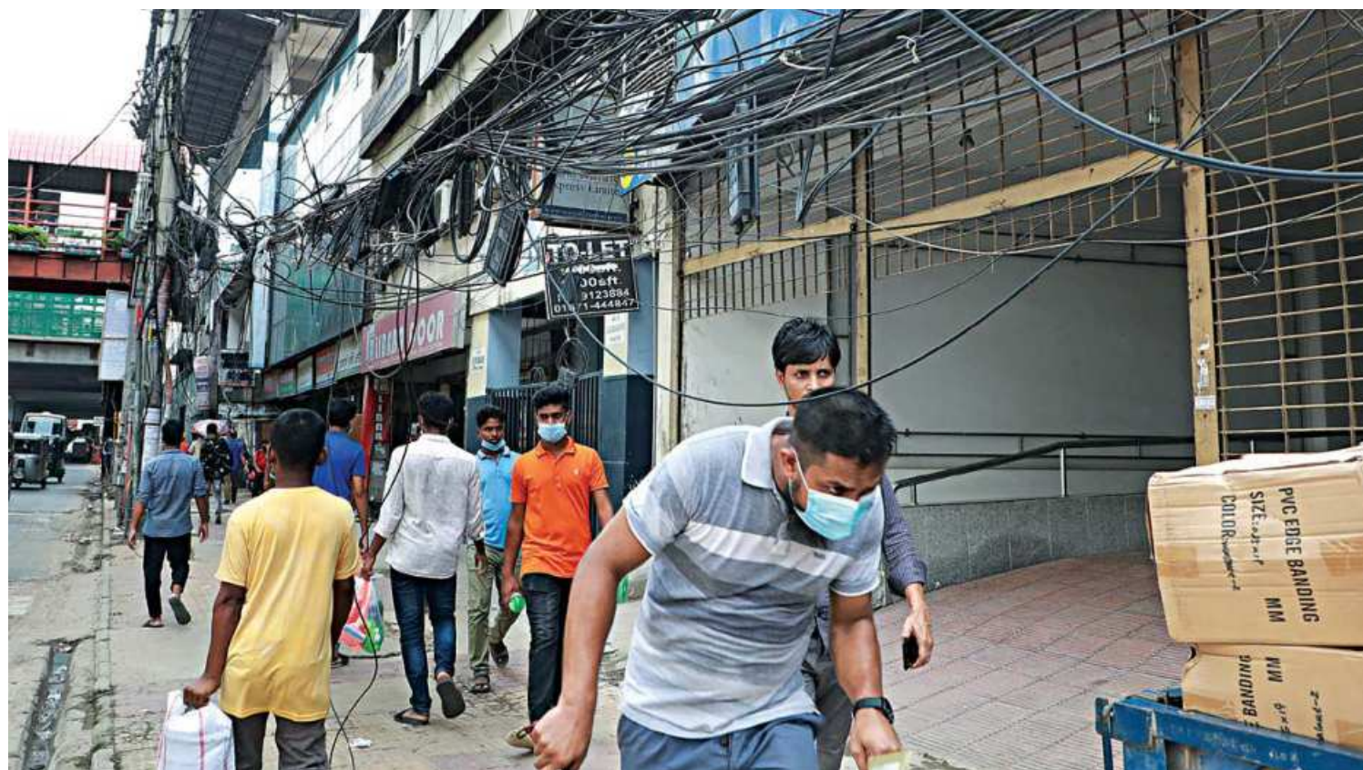
AN OBSTACLE COURSE NO ONE ASKED FOR... Dangling electric, telephone, and internet cables have been around for so long that citizens have become desensitised to them. But ever so often, one will come off the entanglement and hang low, causing a significant but barely noticed hassle for commuters passing by, along with the electrocution risk that comes with it. On top of this, other obstacles on footpaths, like the loaded pickup-van pictured on the right, cause additional difficulty for pedestrians. This photo was taken from the capital's Kazi Nazrul Avenue near Karwan Bazar yesterday.
