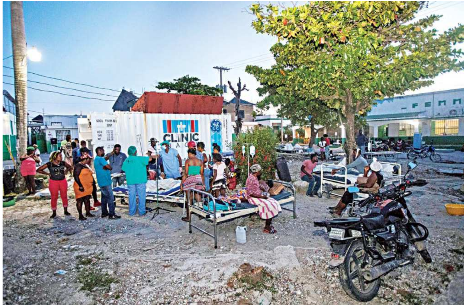
Patients accompanied by their relatives are seen outside a hospital damaged following a 7.2 magnitude earthquake in Les Cayes, Haiti on Saturday.
