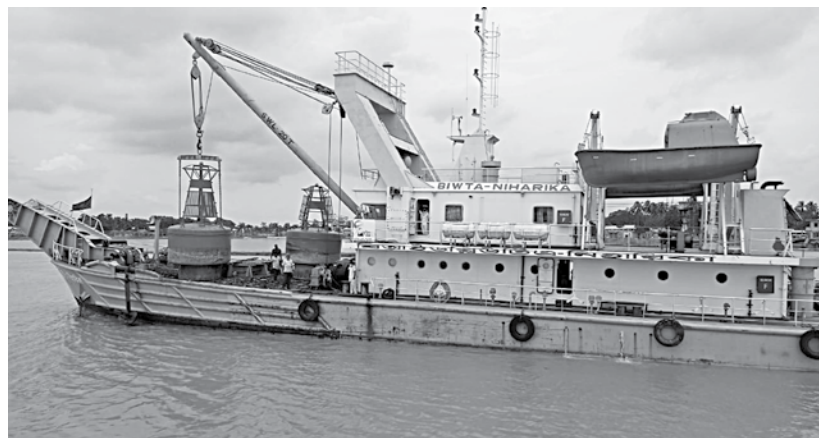
A BIWTA vessel carries the lighted buoy before placing it near Padma Bridge span 12 and 13.
