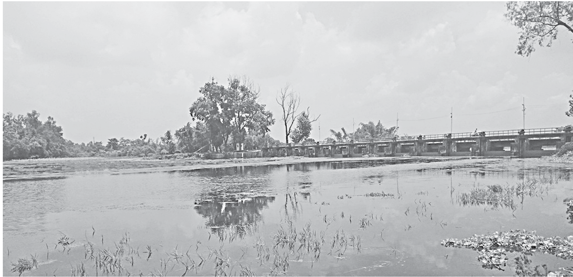
A recent view of the 91-meter-long Buri Teesta barrage and a section of the 1,200-acre water reservoir, which are integral parts of the newly revived irrigation scheme on the Buri Teesta river. The scheme will initially facilitate irrigation facilities for four thousand acres of croplands in Jaldhaka and Dimla upazilas of Nilphamari.
