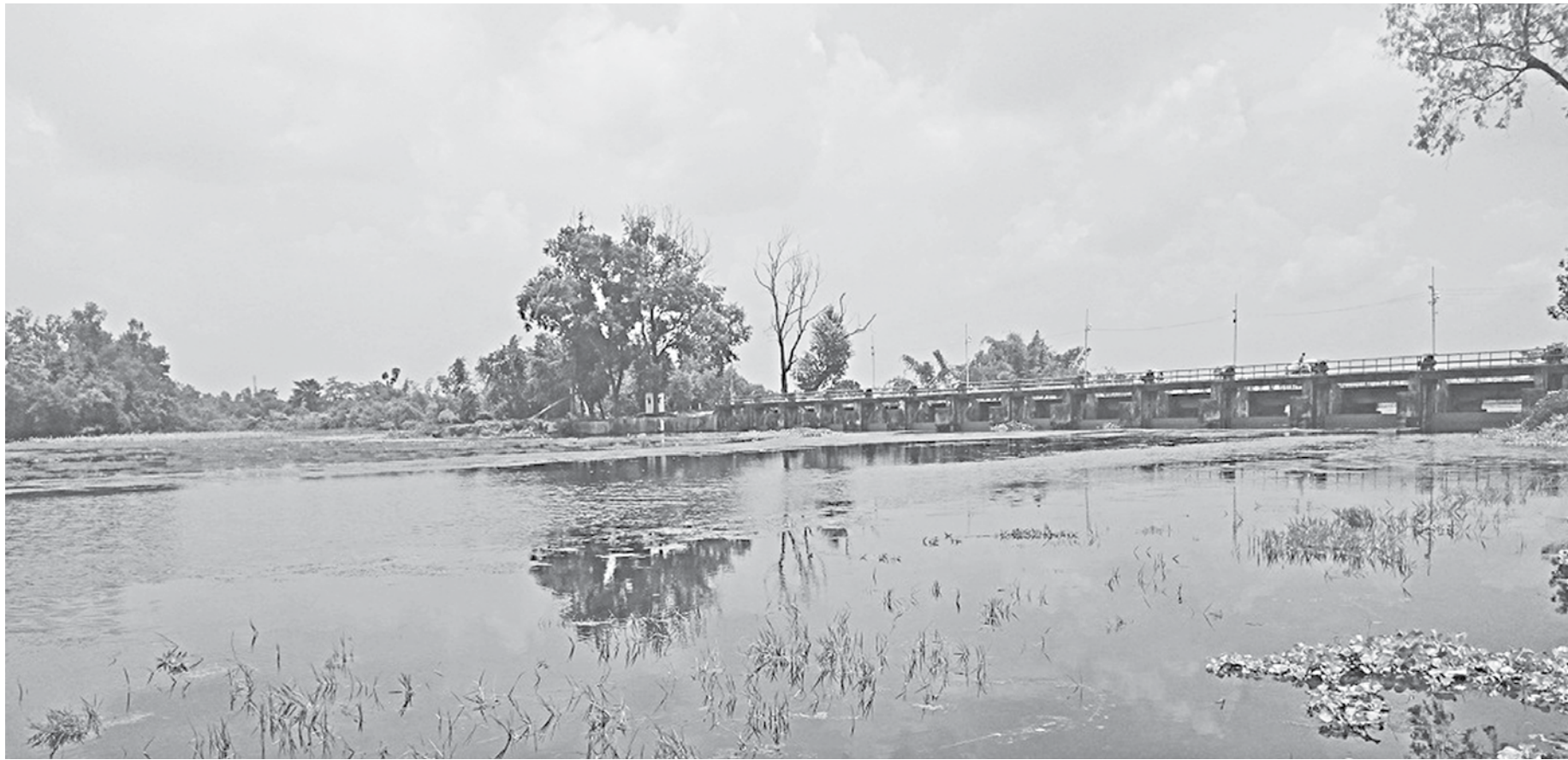
A recent view of the 91-meter-long Buri Teesta barrage and a section of the 1,200-acre water reservoir, which are integral parts of the newly revived irrigation scheme on the Buri Teesta river. The scheme will initially facilitate irrigation facilities for four thousand acres of croplands in Jaldhaka and Dimla upazilas of Nilphamari.
