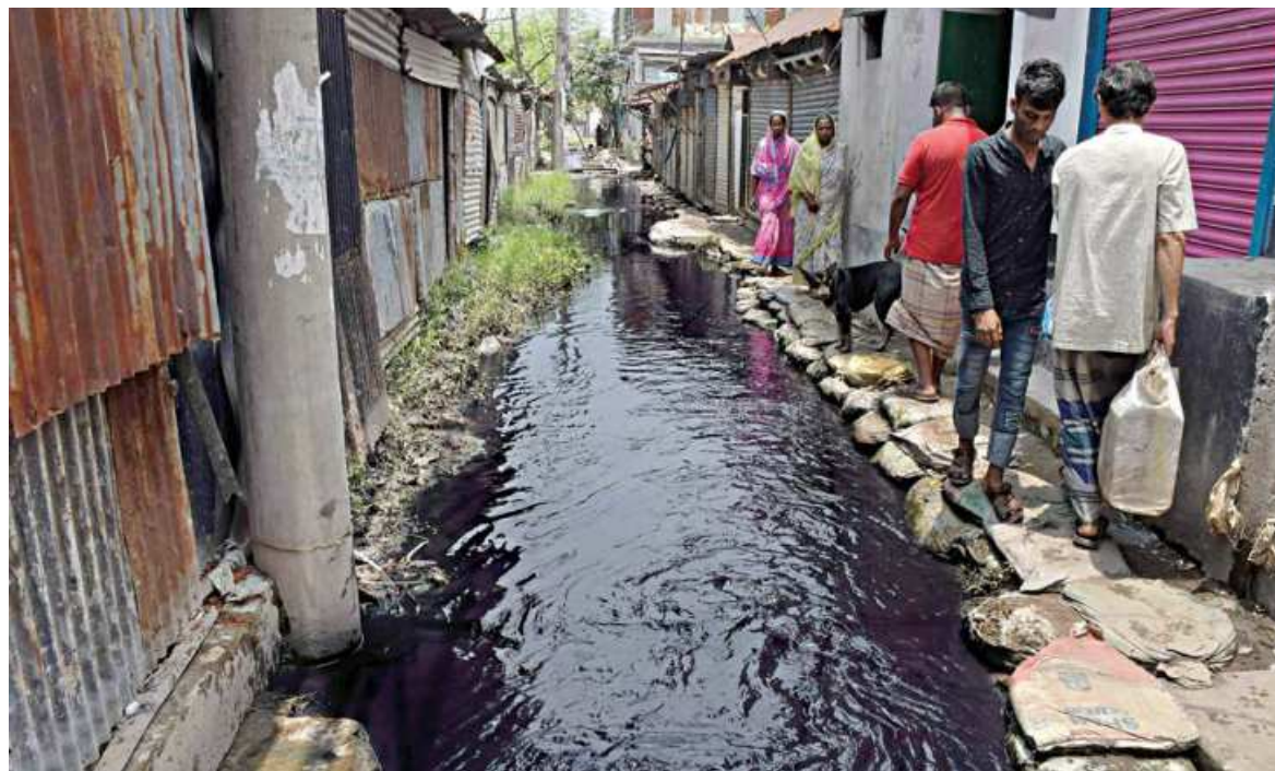
Locals walking on sand bags propped against the edge of a building to avoid the waterlogged pathway in Pagar Alerteg area adjacent to the Tongi Industrial Zone of the Bangladesh Small and Cottage Industries Corporation. Rain causes the area to become flooded by pitch-black filthy water from the nearby factories. The photo was taken recently.
