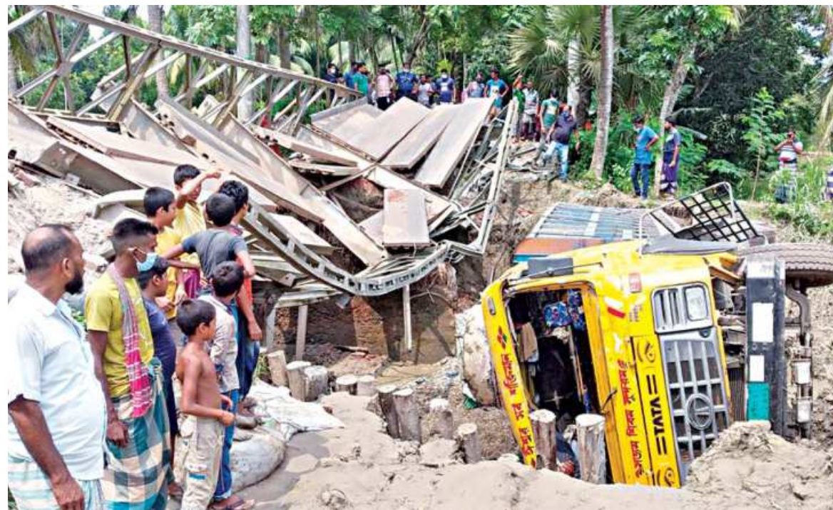
A stone-laden truck lies on its side in a canal in Shariatpur yesterday after the Bailey bridge, not designed to carry so much weight, collapsed. Most Bailey bridges were built on temporary basis with a standard load capacity of 7.50 tonnes.
