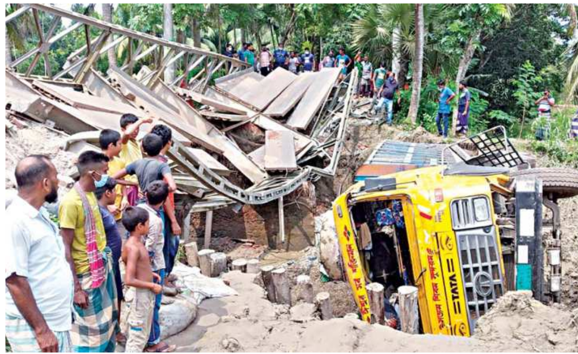
A stone-laden truck lies on its side in a canal in Shariatpur yesterday after the Bailey bridge, not designed to carry so much weight, collapsed. Most Bailey bridges were built on temporary basis with a standard load capacity of 7.50 tonnes.
