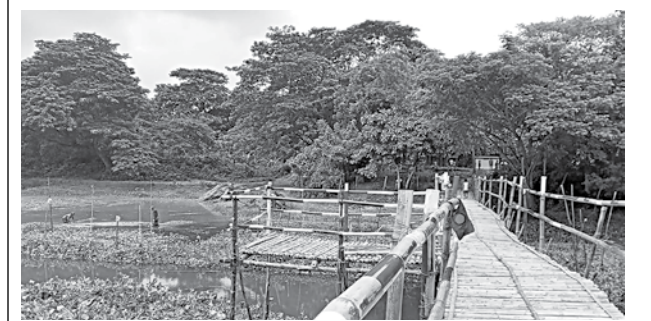
The bamboo and wooden bridge has connected seven villages in Kaliganj upazila of Jhenidah easing the movement of the villagers.
