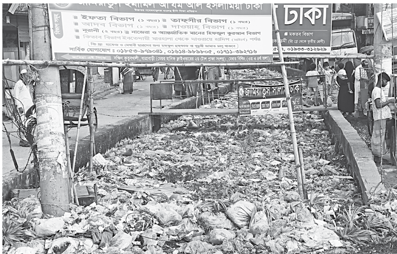
Once part of Jatrabari's Kutubkhali canal, this waterbody has been turned effectively into a large gutter due to construction work around it and then filled up with waste to the point no water passes through it. Only a few months ago, Dhaka South City Corporation had cleaned it up, but that effort has gone down the proverbial drain, judging by the looks of it. The photo was taken yesterday.
