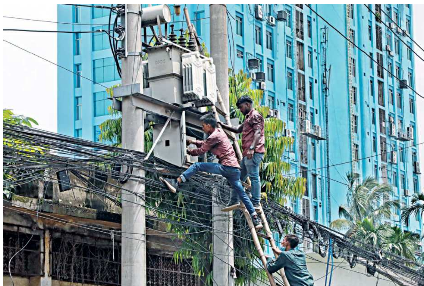
With one foot on the ladder and the other resting precariously on wires, an electrician along with his workmates is busy working on a transformer. One misstep at any point of the work may lead to a serious accident. This photo was taken yesterday from the capital's Tejjanga.
