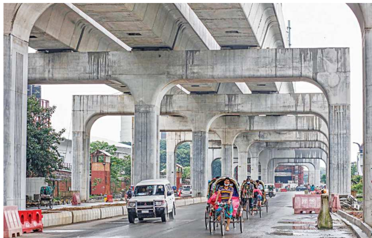
As the metro rail is 68 percent towards completion, some roads of the capital have regained their space for vehicular movement, as it was lost due to construction materials and machineries occupying large parts of the roads. This photo was taken from the capital's Sher-e-Bangla Nagar area on Monday.
