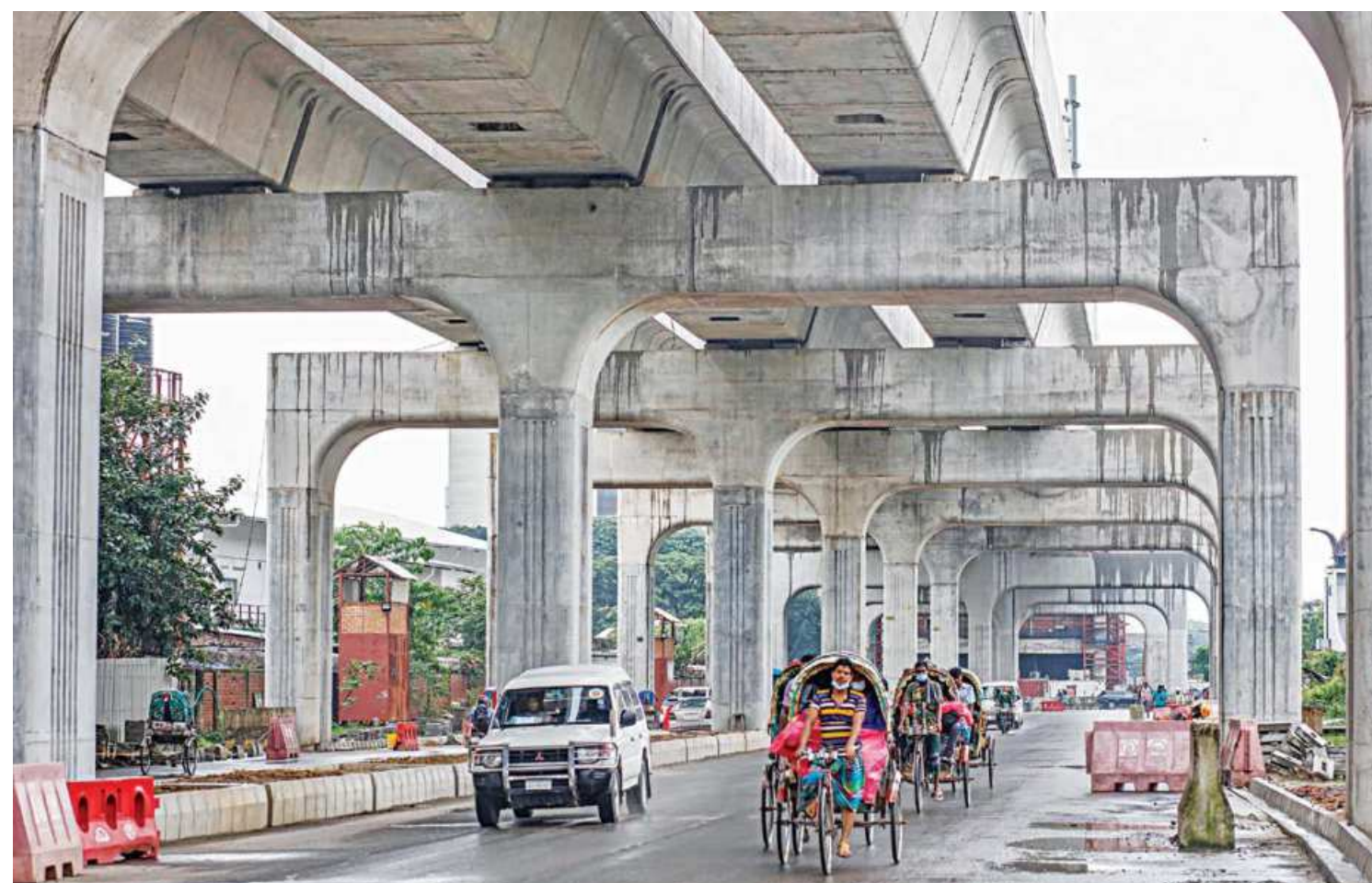
As the metro rail is 68 percent towards completion, some roads of the capital have regained their space for vehicular movement, as it was lost due to construction materials and machineries occupying large parts of the roads. This photo was taken from the capital's Sher-e-Bangla Nagar area on Monday.
