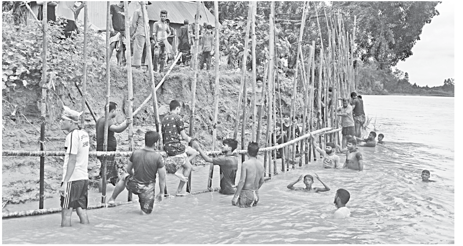
Locals join voluntary service to construct an embankment on Louhajang river to save an Eid congregation ground, a graveyard and a dakhil madrasa from erosion.
