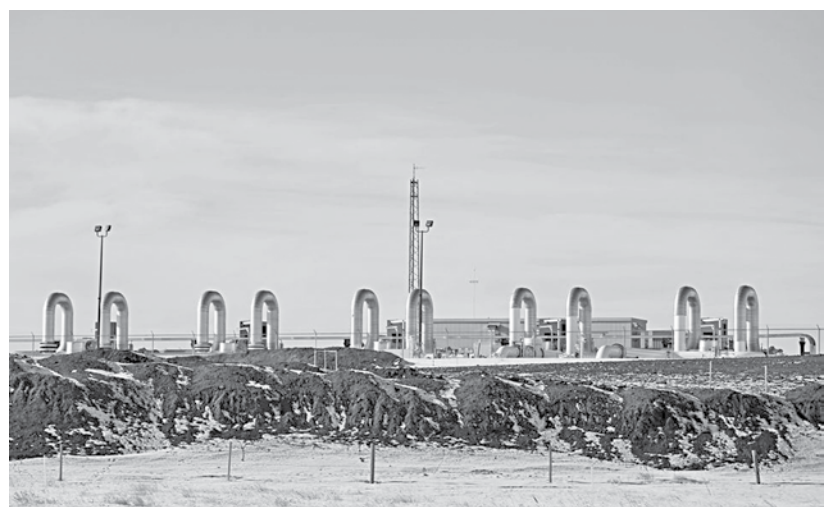
A TC Energy pump station sits behind mounds of dirt from the Keystone XL crude oil pipeline as it lies idle near Oyen, Alberta, Canada on February 1.
