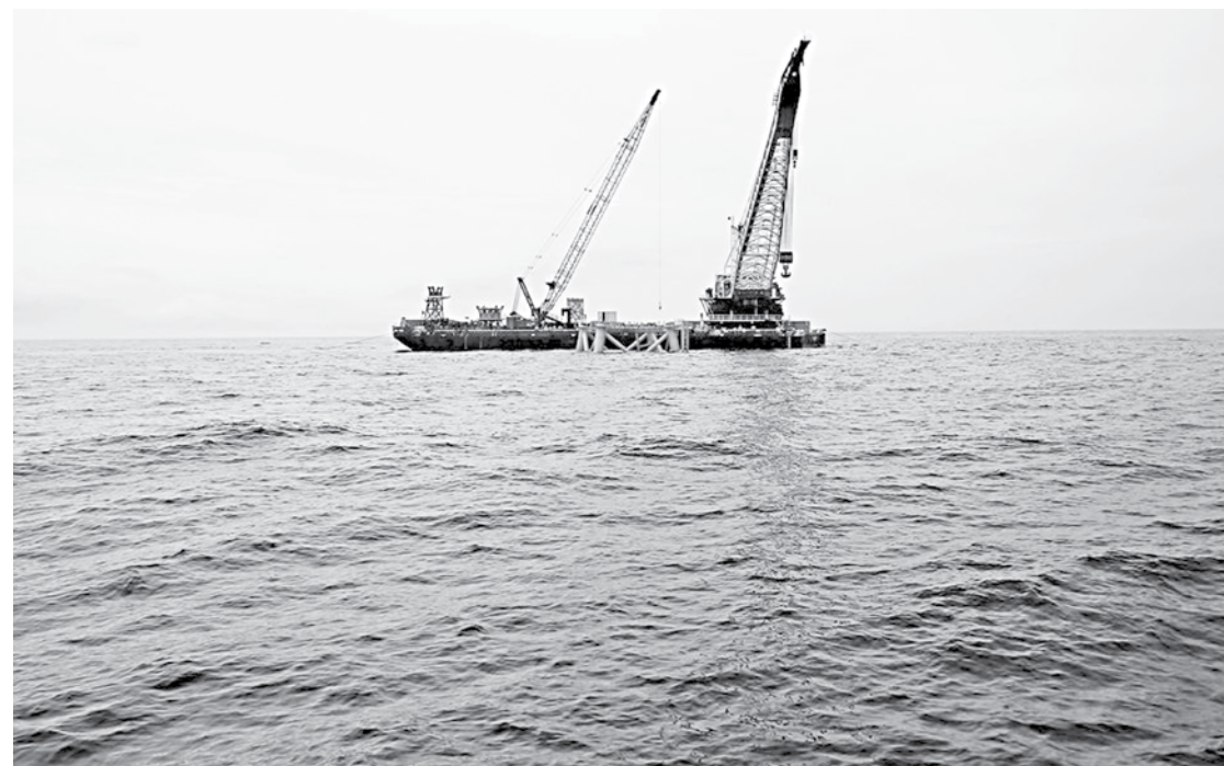
A crane hangs over the first jacket support structure installed to support a turbine for a wind farm in the waters of the Atlantic Ocean off Block Island, Rhode Island.
