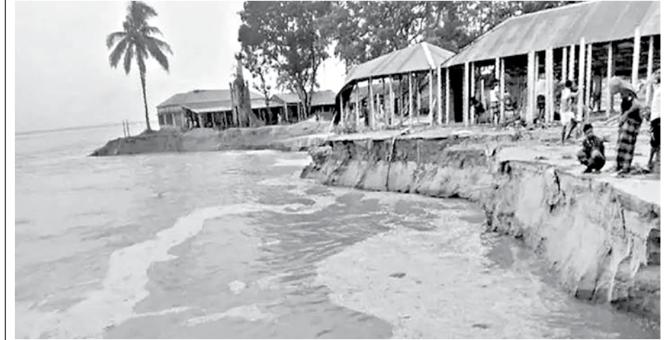
A view of erosion affected Durgapur area in Tangail's Kalihati upazila.
