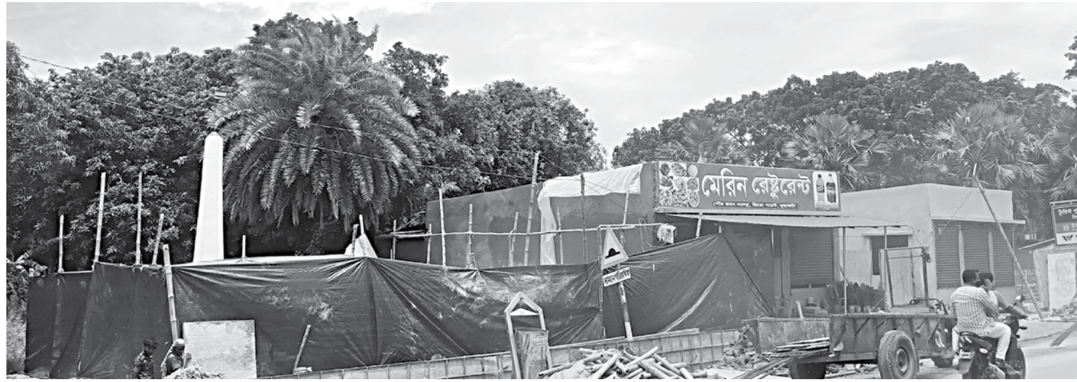
Concealed behind polythene sheets, construction of shops is underway on Patuakhali-Kuakata highway near Kuakata Municipality building. The structures under construction and the ones already built are on the land that belongs to a two hundred year-old Buddhist temple (visible behind the polythene covering), monastery and graveyard of Rakhine community.
