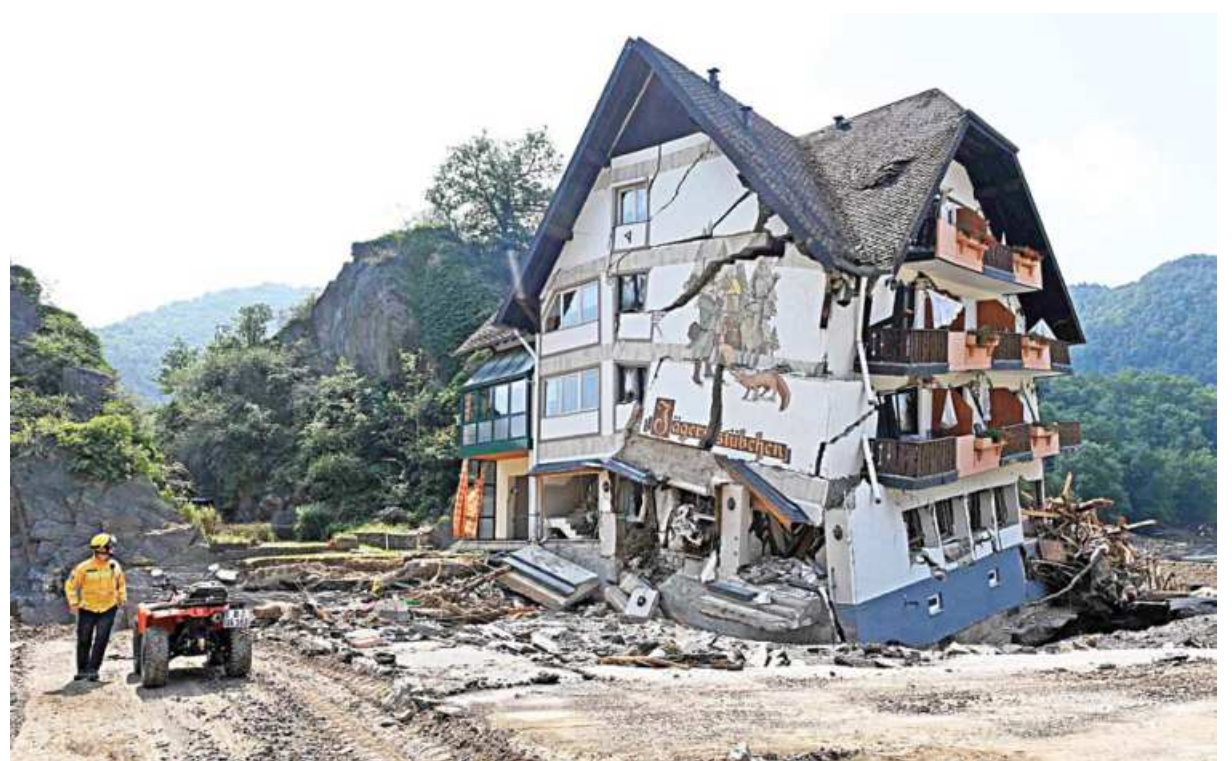
A man walks in front of a destroyed building in Laach, part of the municipality of Mayschoss, district of Ahrweiler, western Germany, on Friday, about a week after floods caused major damage in the Ahr region. The latest death toll from floods that hit western Germany this month stands at 180, with about 150 still missing, authorities said. PHOTO: AFP
