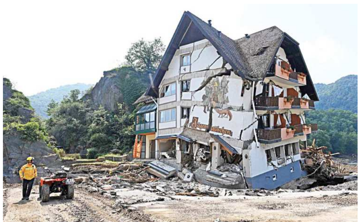
A man walks in front of a destroyed building in Laach, part of the municipality of Mayschoss, district of Ahrweiler, western Germany, on Friday, about a week after floods caused major damage in the Ahr region. The latest death toll from floods that hit western Germany this month stands at 180, with about 150 still missing, authorities said. PHOTO: AFP
