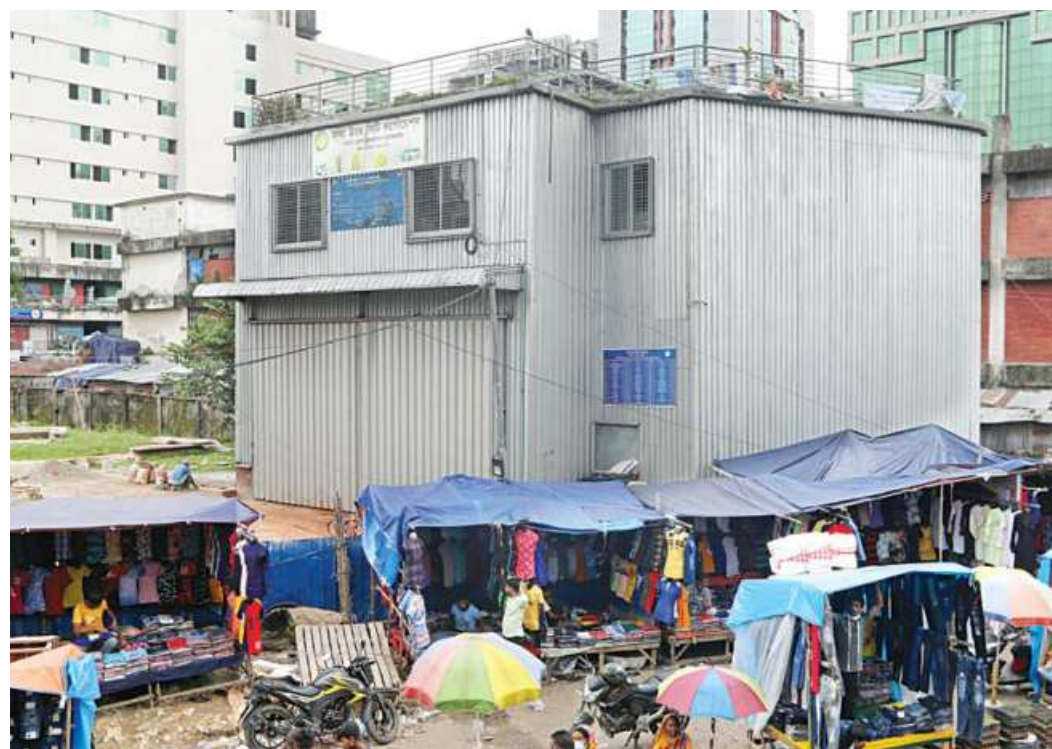
An emergency response warehouse of Dhaka North City Corporation in the capital's Karwan Bazar. Different types of imported firefighting equipment have been gathering dust at the warehouses of city corporations as those remain unused for about one and a half years. Top right, a generator at the emergency response warehouse at Mirpur-10. Bottom right, a server at Mohakhali satellite control room.
