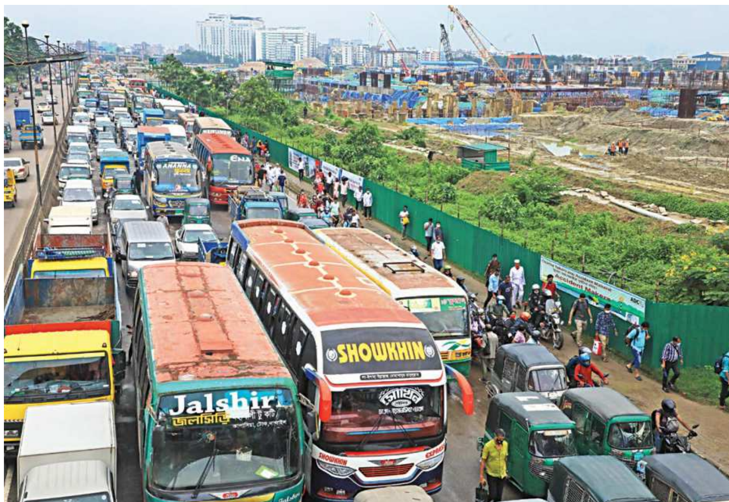
Due to rain and the Eid rush, heavy traffic ran from Banani all the way to Tongi bridge. Many roads along the route remained gridlocked from morning to late afternoon. The photo was taken at Kawla bridge near the airport.
