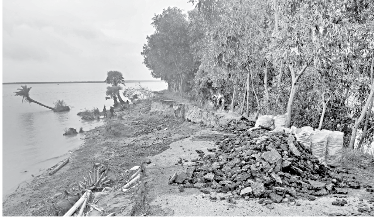
Nearly twenty thousand inhabitants of at least eight villages in Patuakhali's Dashmina upazila have been suffering immensely since this road, built on the flood control dyke along the Tentulia river, washed away by the cyclone Yaas.
