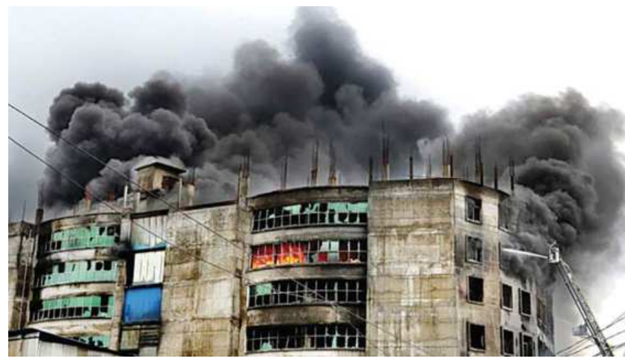
Smoke billows from the six-storey factory building of Hashem Foods as firefighters try to put out the flames on July 9.
