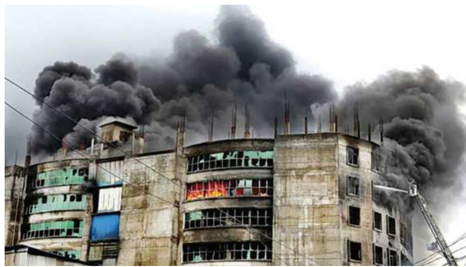
Smoke billows from the six-storey factory building of Hashem Foods as firefighters try to put out the flames on July 9.
