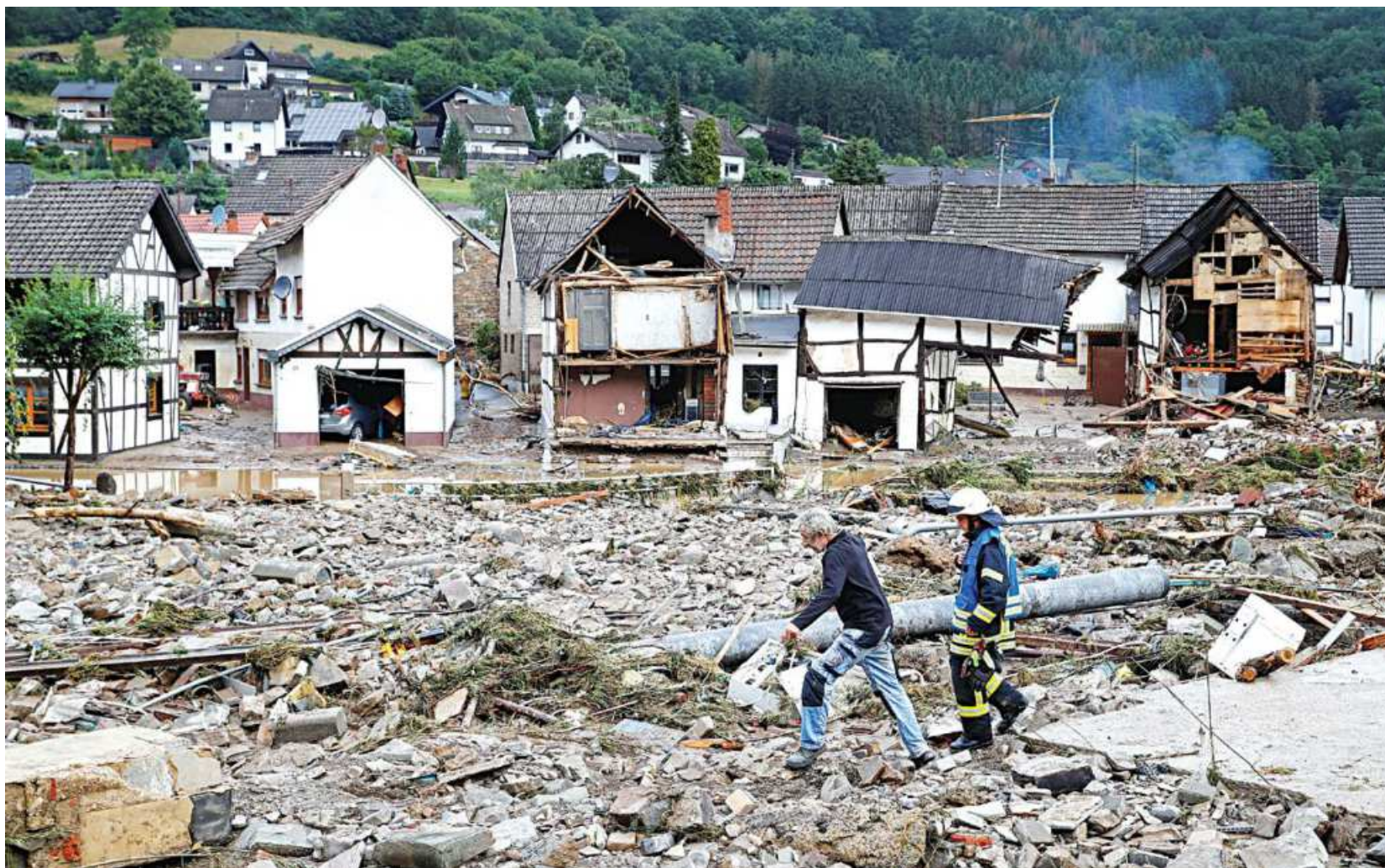
Rescue workers walk through debris, following heavy rainfalls in Schuld, Germany, yesterday. Heavy rains and floods lashing western Europe have killed at least 42 people in Germany and left many more missing, as rising waters led several houses to collapse yesterday. Unusually heavy rains also inundated neighbouring Luxembourg, the Netherlands and Belgium, where at least four people were reported dead.
