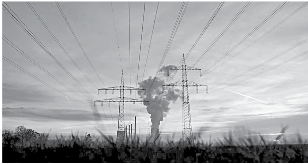
General view of electricity pylons and power lines leading from the Uniper coal power plant in Hanau, Germany.
