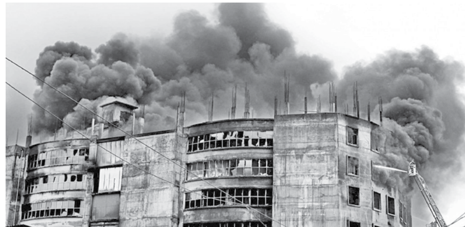
Smoke billows from the six-storey factory building of Hashem Foods as firefighters try to put out the flames on July 9, hours after a fire broke out at the factory in Karmagop area of Narayanganj's Rugganj upazila.
