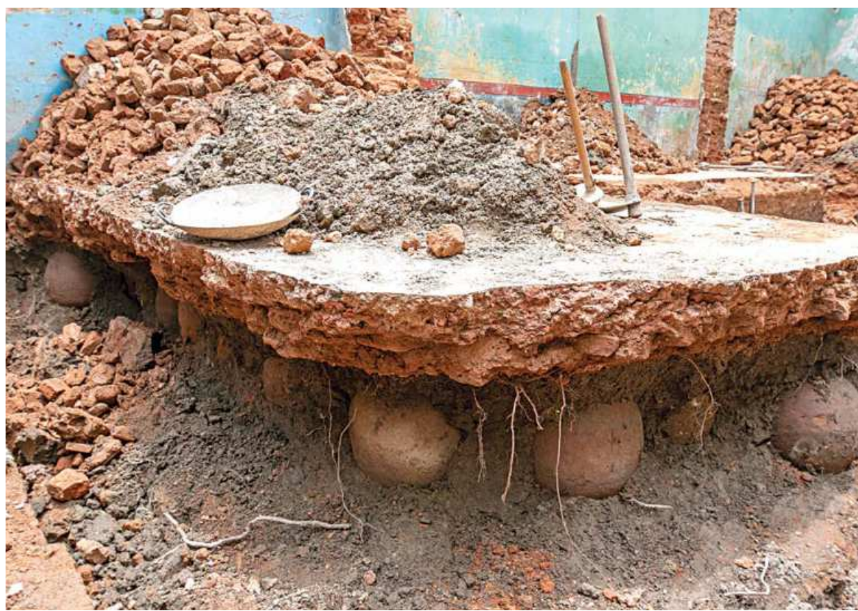
After dismantling part of the basement of a 300-year-old one-storey building, these clay pots were found to be supporting the whole structure, which fascinated locals. Over a hundred of these egg-shaped pots are bearing the weight of around 2,500 tonnes. Experts say the technology was used during the Mughal era to manage temperature of buildings and make them resistant to earthquakes and flood. The photos were taken yesterday.
