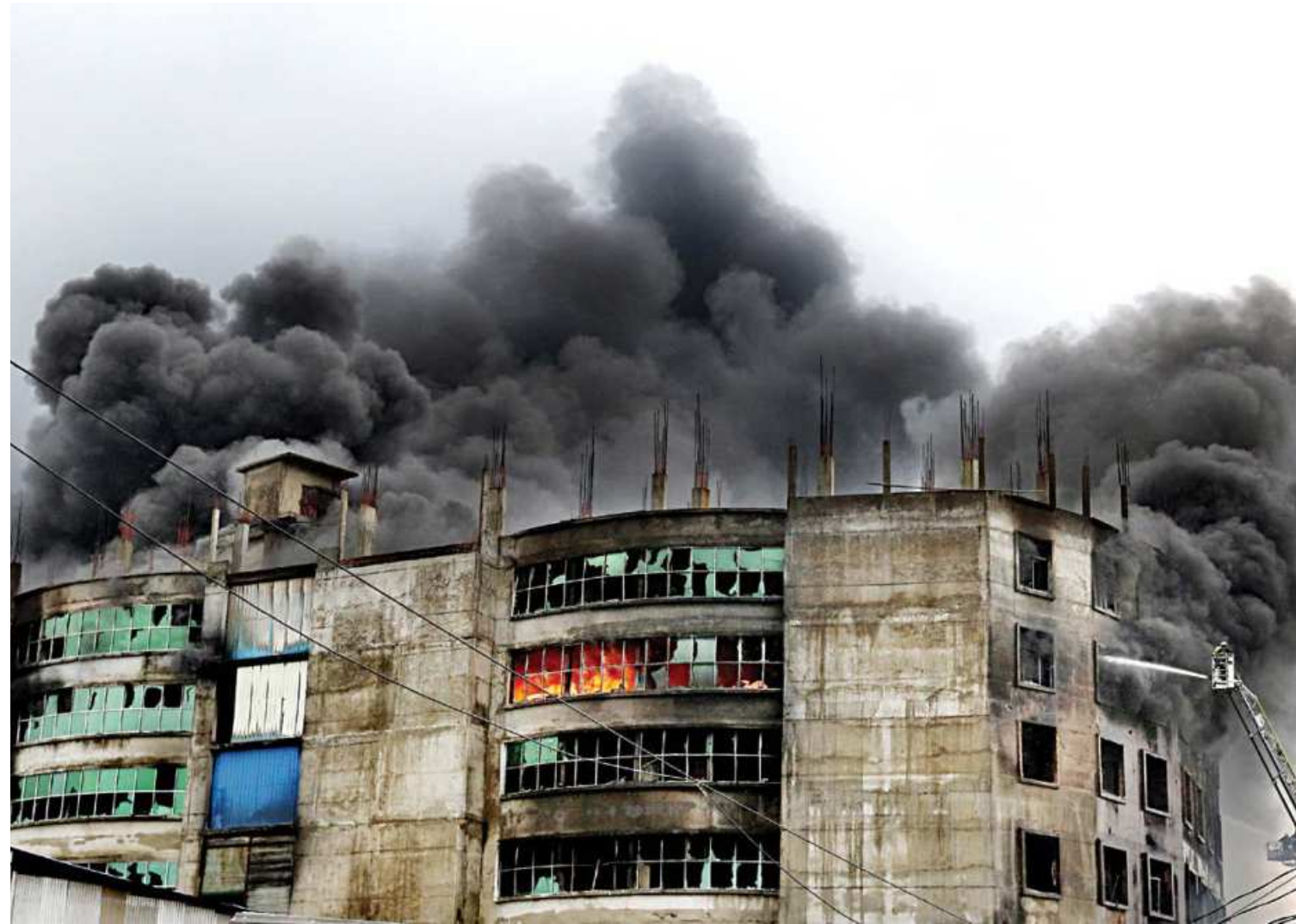
Smoke billows from the six-storey factory building of Hashem Foods as firefighters try to put out the flames yesterday, hours after a fire broke out at the factory in Karnagop area of Narayanganj's Rugganj upazila. The massive blaze swept through the building, leaving at least 52 people dead. More photos on page 3.
