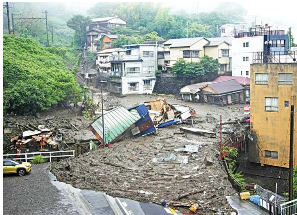
Houses damaged by a mudslide are seen following heavy rain in Izusan district in Atami, Japan, yesterday. At least two people were feared dead after landslides triggered by heavy rains hit the central Japanese city of Atami, where about 20 people were still missing, public broadcaster NHK said.
