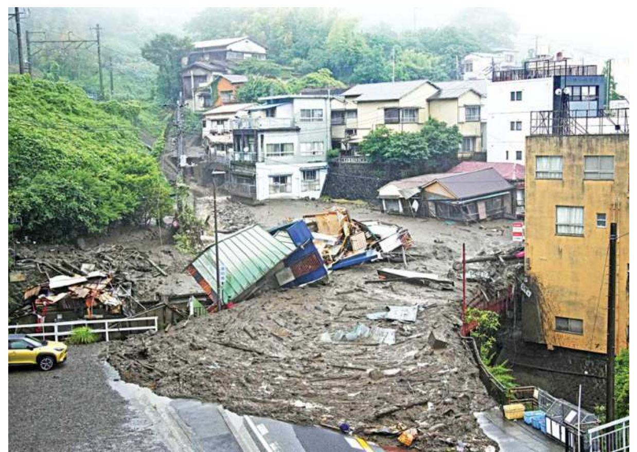
Houses damaged by a mudslide are seen following heavy rain in Izusan district in Atami, Japan, yesterday. At least two people were feared dead after landslides triggered by heavy rains hit the central Japanese city of Atami, where about 20 people were still missing, public broadcaster NHK said.
