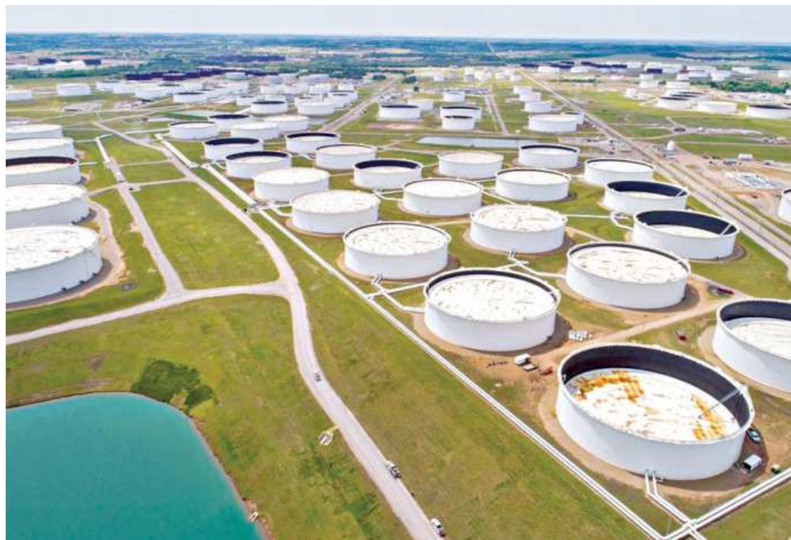
Crude oil storage tanks are seen in an aerial photograph at the Cushing oil hub in Cushing, Oklahoma, US on April 21, 2020.
