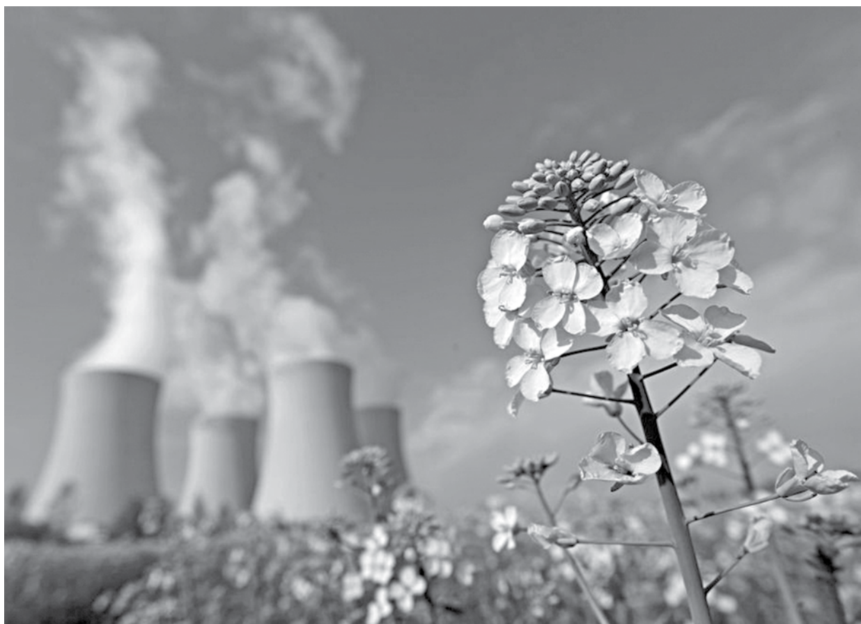
A mustard field is seen in front of the cooling towers of the Temelin nuclear power plant near the South Bohemian city of Tyn nad Vitavou, Czech Republic.
