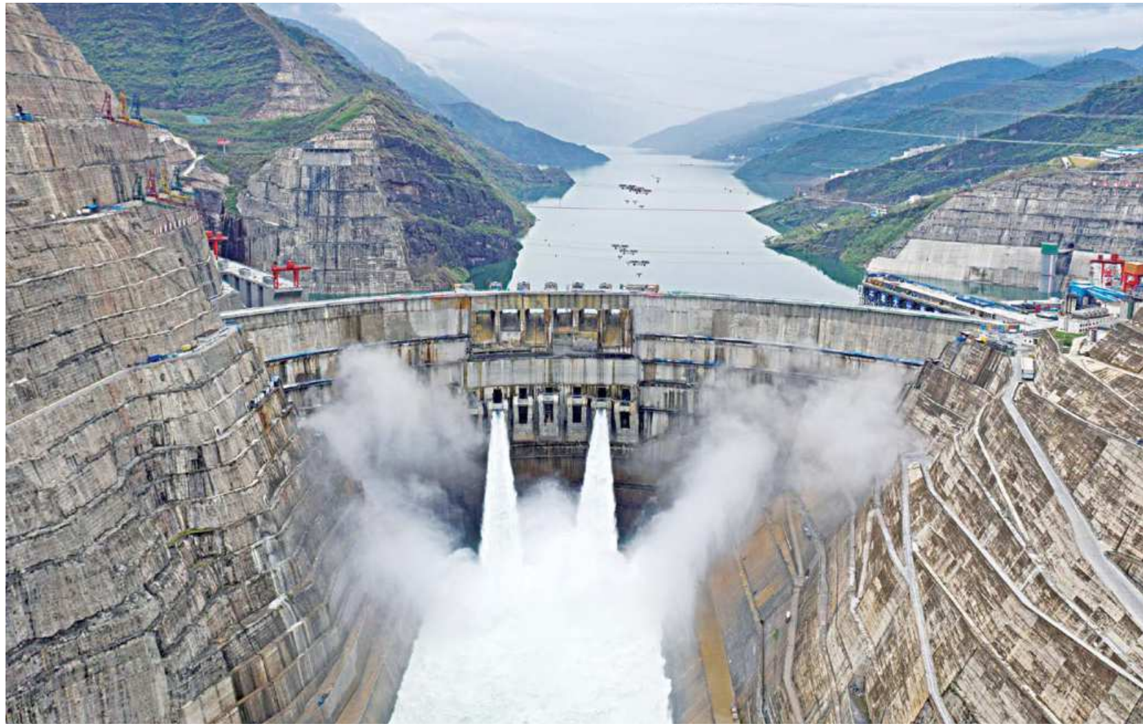
The Baihetan hydropower plant is seen in operation on the border between Qiaojia county of Yunnan province and Ningnan county of Sichuan province, yesterday. The 289-metre (948 feet) high Baihetan Hydropower Station in southwest China, second in the world only to the country's Three Gorges Dam in terms of power generation, began partial operation yesterday morning, state media reported. Baihetan was built with a total installed capacity of 16,000 megawatts.
