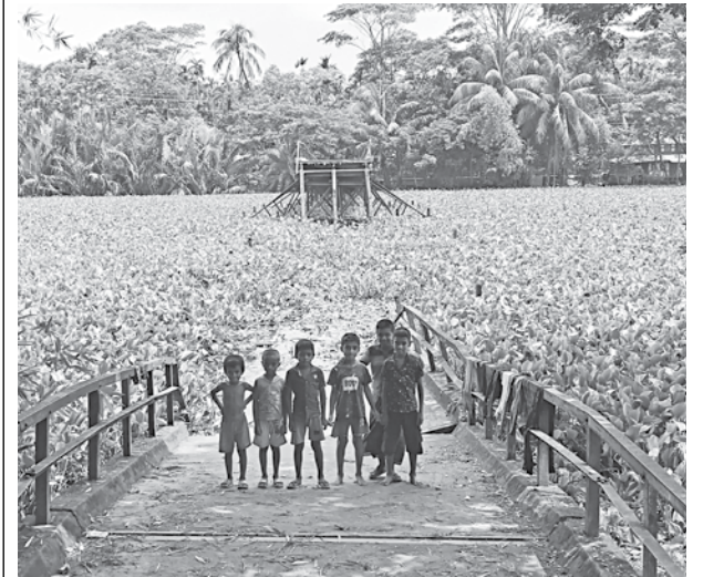
The bridge on Chawra canal, in Mohishdanga area of Barguna's Amtali upazila, collapsed on June 25.
