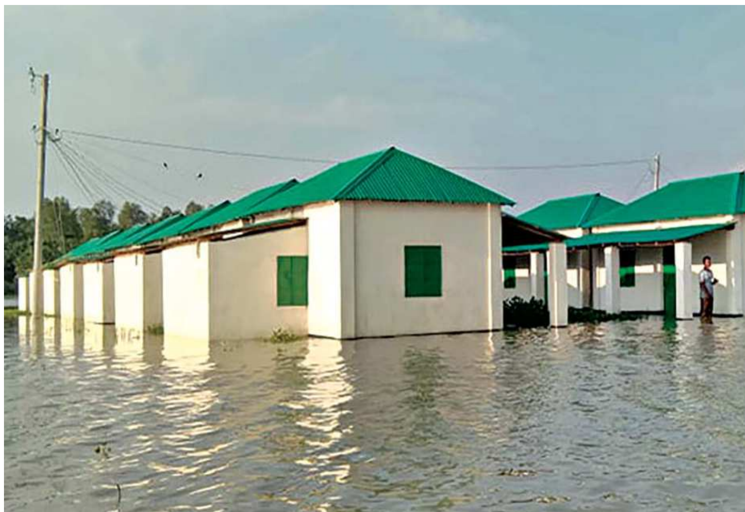
Houses built under the Ashrayan-2 project, which gives houses to landless and homeless families, in Jamalpur's Sarishabari upazila have been flooded during monsoon. Twenty-one families who received the houses recently are currently displaced due to the flooding. The photo was taken on Wednesday.
