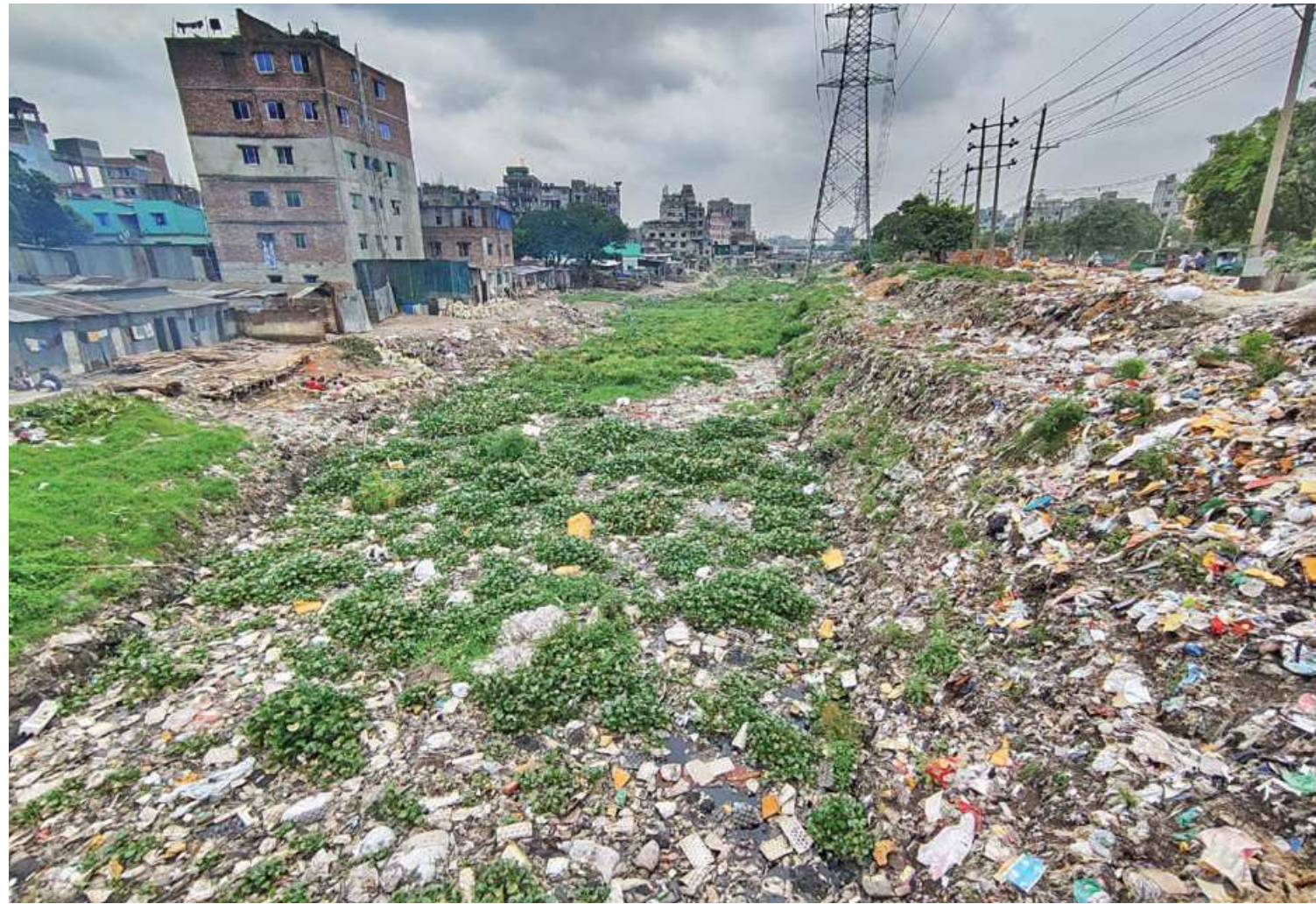
Hard to imagine that this is actually a canal meant for draining storm water out. Excavation of the canal had started but it was not completed. The photo was taken near Kamrangirchar in Dhaka.
