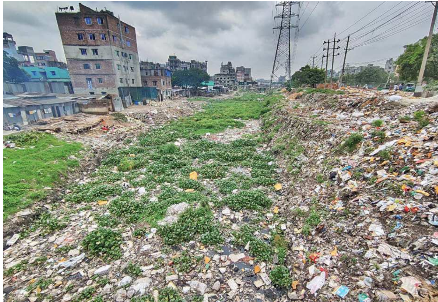
Hard to imagine that this is actually a canal meant for draining storm water out. Excavation of the canal had started but it was not completed. The photo was taken near Kamrangirchar in Dhaka.
