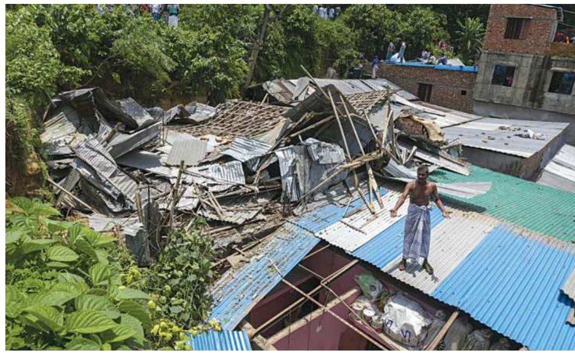
A man stands on the roof of his torn down house after Chattogram district administration evicted people living on the hill slopes ignoring risks of landslides. The photo was taken in Lal Khan Bazar of the port city.
