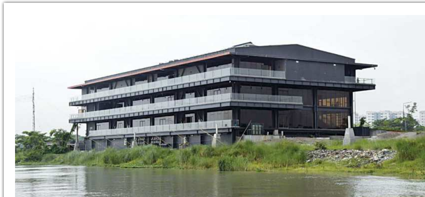
A view of Dhaka Boat Club on the Turag river in Birulia. The club was set up allegedly on the flood-flow zone along the Dhaka flood protection embankment. The photo was taken last week.
