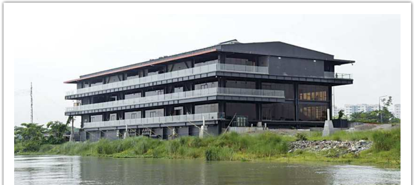
A view of Dhaka Boat Club on the Turag river in Birulia. The club was set up allegedly on the flood-flow zone along the Dhaka flood protection embankment. The photo was taken last week. PHOTO: STAR
