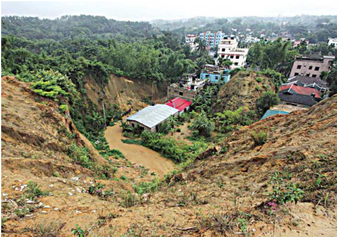
Risking their lives, people living on the slopes of hills in Sylhet city's Nayabazar Kalibari area. Heavy rain may trigger fatal landslides. This photo was captured recently.
