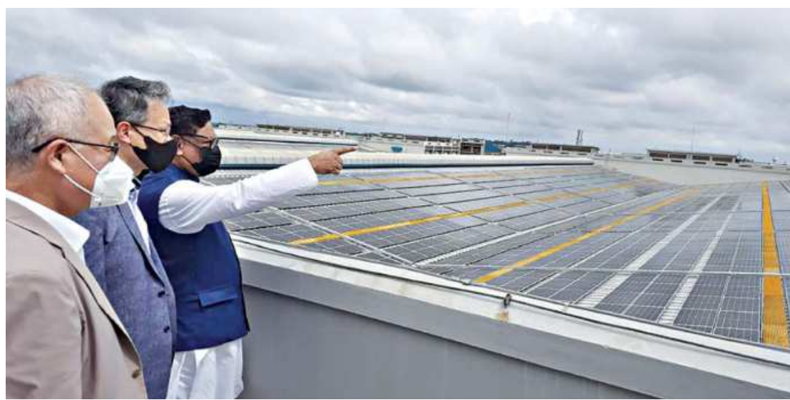
State Minister for Power Nasrul Hamid is seen visiting Youngone Corporation's rooftop solar plant along with Korean Ambassador Lee Jang-Keun and Youngone Chairman Kihak Sung in Chattogram yesterday.
