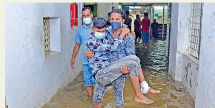
Agrabad's Ma O Shishu Hospital is a regular victim of waterlogging in the city, and yesterday was no exception. The situation was so bad that patients had to be carried through the entrance by their relatives.
