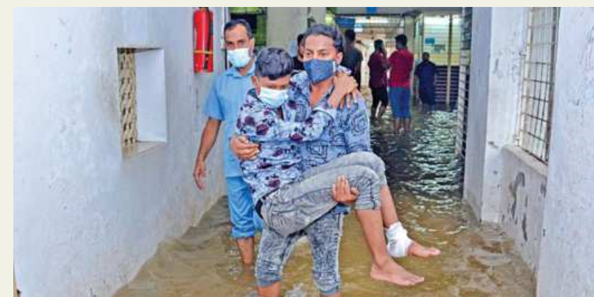
Agrabad's Ma O Shishu Hospital is a regular victim of waterlogging in the city, and yesterday was no exception. The situation was so bad that patients had to be carried through the entrance by their relatives.
