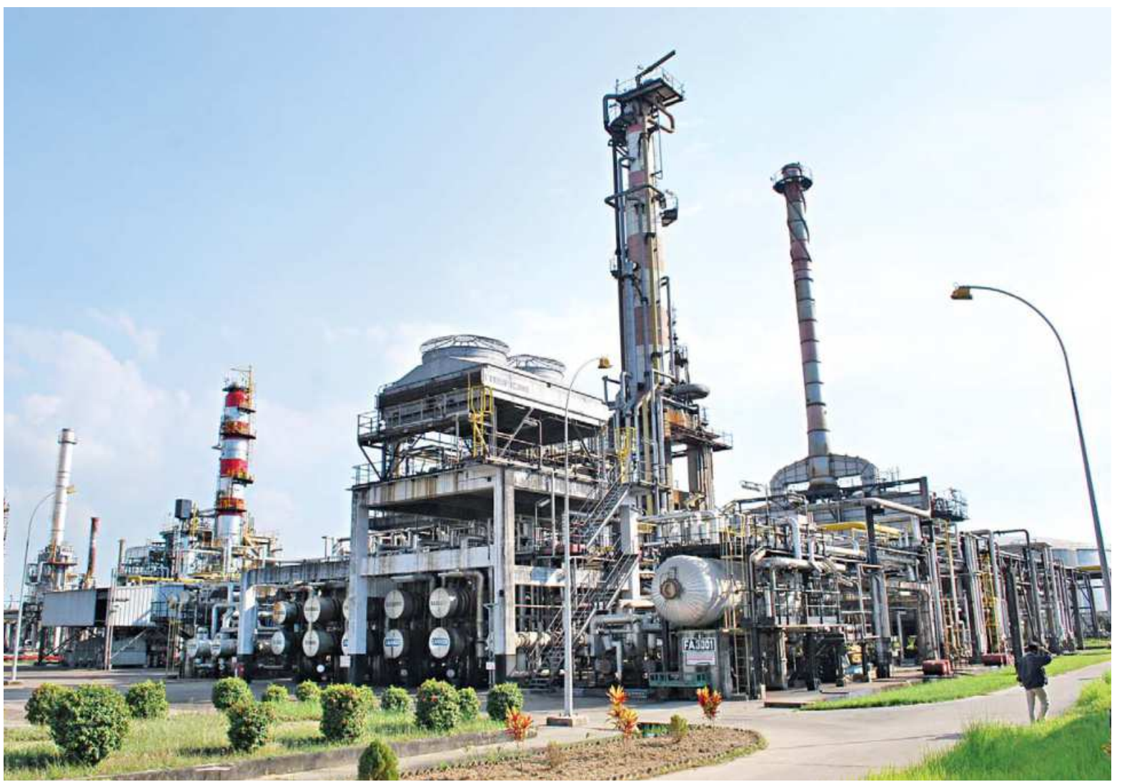
The lone unit of state-run Eastern Refinery in Chattogram was commissioned in 1968. The economic life of the plant was estimated to be 20 to 25 years. Today, it refines 12 lakh tonnes of crude oil annually against the capacity of 15 lakh tonnes. The photo was taken earlier this year.
