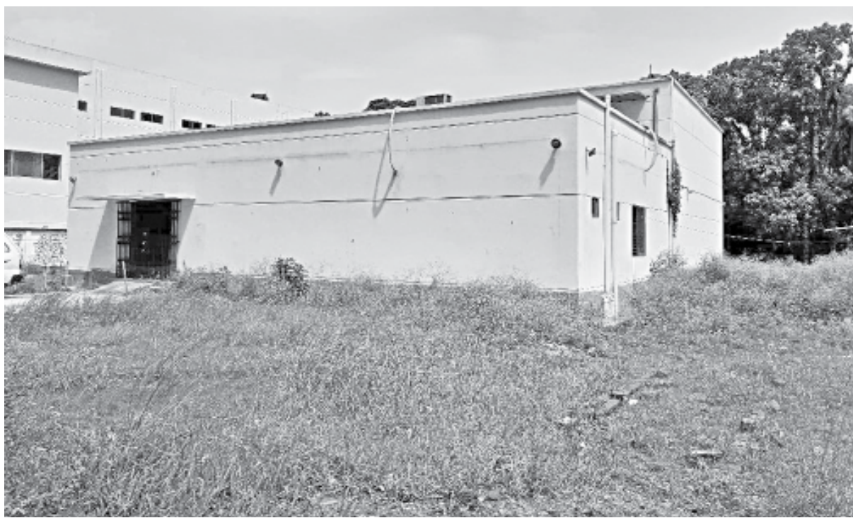
Grass is growing high around the cancer unit building of Bangabandhu Sheikh Mujib Medical College Hospital in Faridpur town -- a sign that the facility is not being maintained properly.
