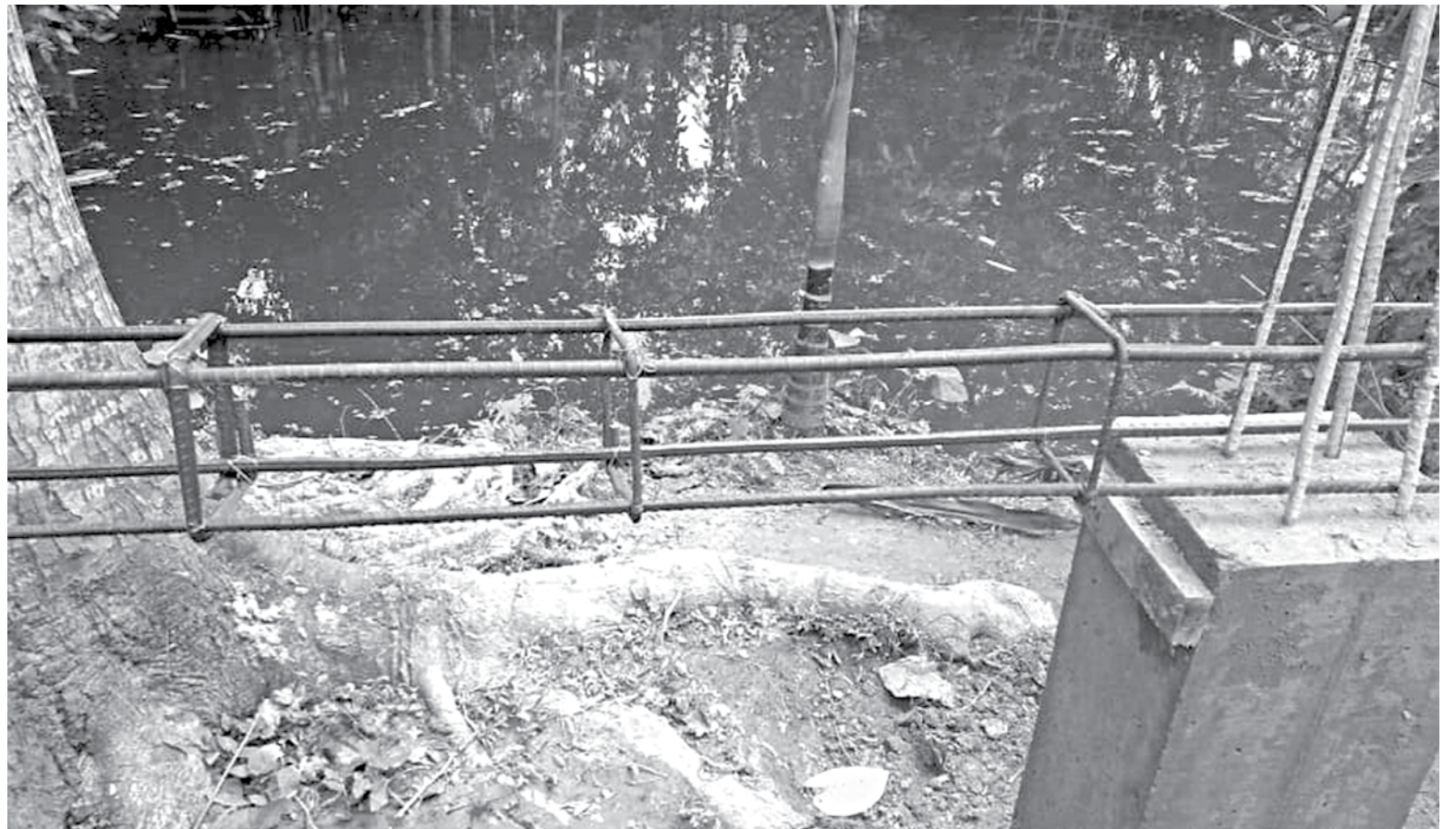
Rebar rings are being used around 15 inches apart from each other in a lintel for the under construction boundary wall of Babur Bazar Government Primary School in Moulvibazar's Rajnagar upazila.
